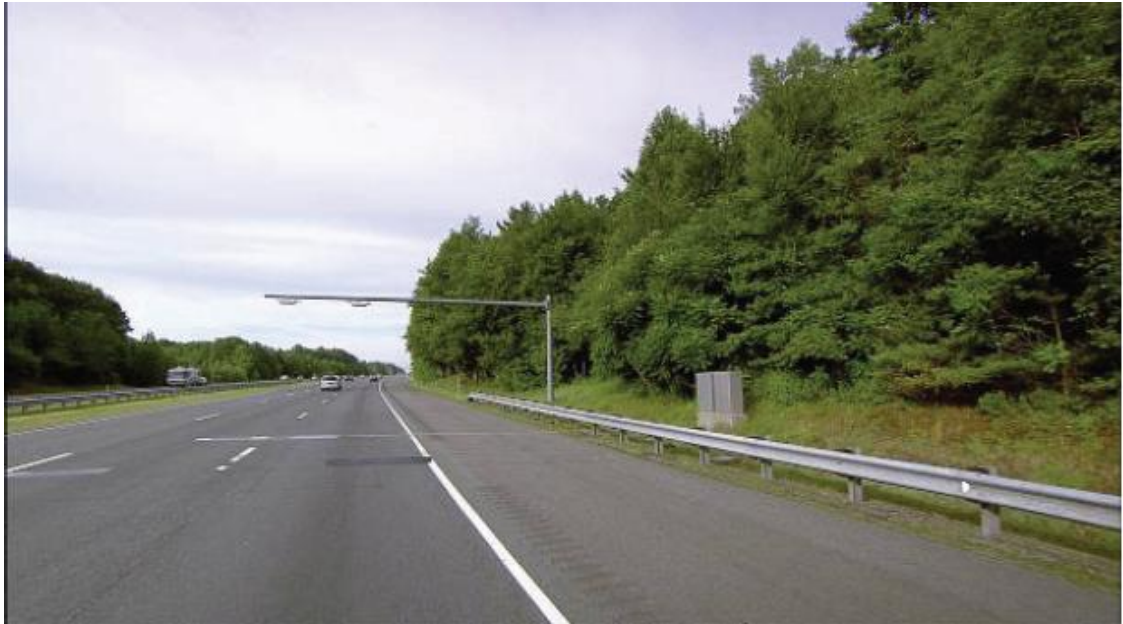
Photograph 4.3: Automated WIM /ANPR in Connecticut, USA
