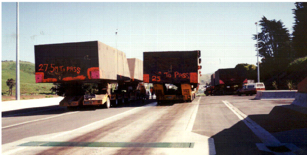
Photo 5.2 Plimmerton Weigh station (showing the dynamic weigh strip and operational requirement for a large parking area).
