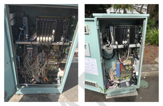
Depending on the existing hardware available at the cabinet, the minimum addition into the cabinet will be a network switch to connect multiple cameras into the network. Uninterruptable Power Supplies could also be considered to provide operation or at minimum a graceful shutdown of systems in case of a power failure.
