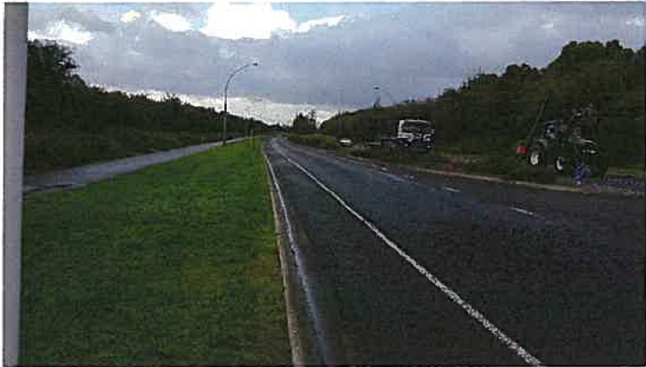
Urban Road (Residential) (Source: G Lane)
